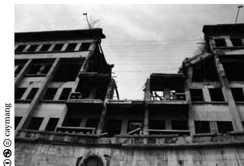
Building in Belgrade bombed by NATO in 1999, Serbia.
